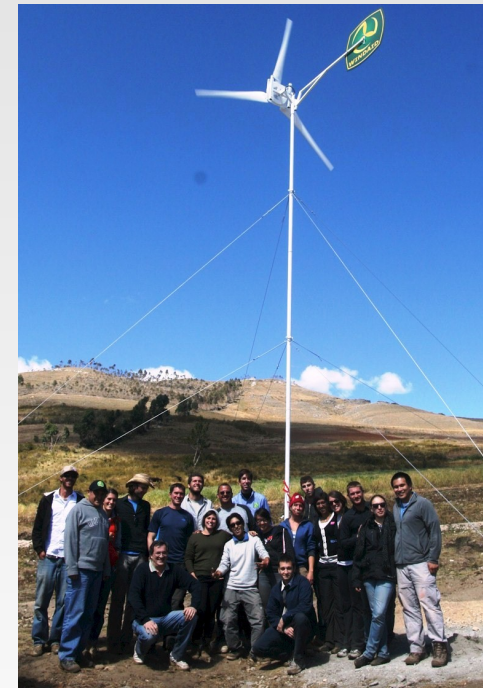
Locally constructed SWT installed - photo Wind Aid Peru
