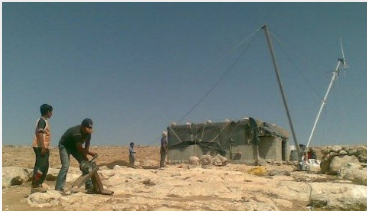
Tilt-up using a gin pole - photo Comet-me Palestaine
